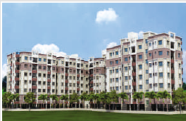
GREEN OASIS - KAIKHALI, KOLKATA
